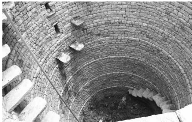
Figure 2. The open wells have dried up in most parts of peninsular India, where borewell pumping has lowered the water table drastically (Photograph by: Kirubakaran Jeremiah)
